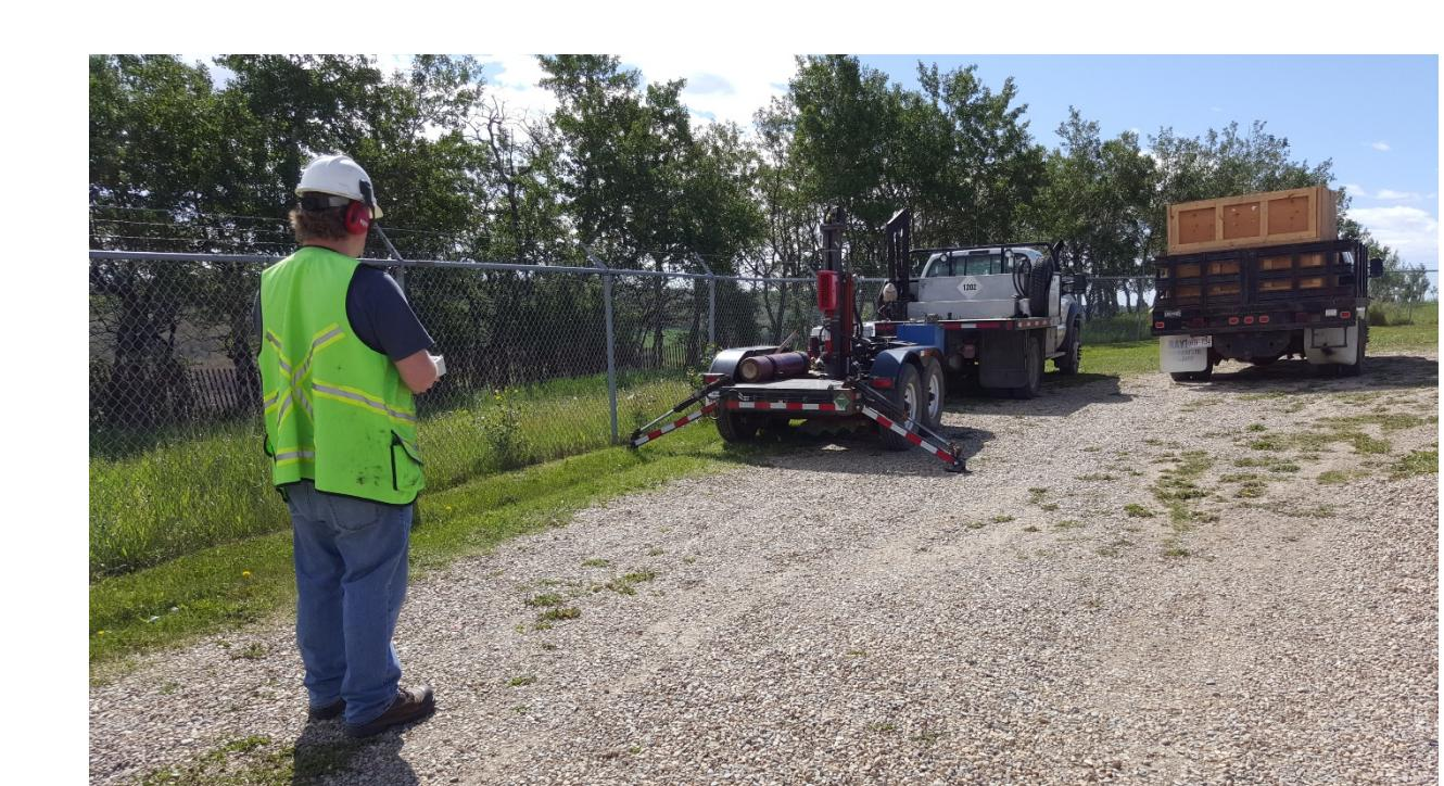
FIG. 9. Operating thumper from a distance.
