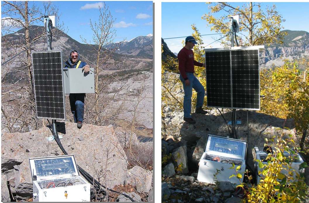
Figure 7. Upgraded power generation system at Pit station. The upgraded system (right) now provides double the generating and storage capacity.
