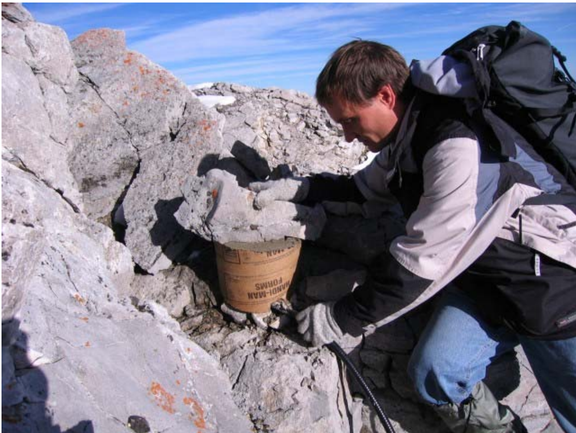
Figure 11. The new geophones are encapsulated by a concrete cylinder. A rock is used to hold the forms in place while the cement cures.
