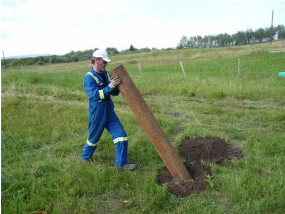
FIG. 9. Casing the shot holes.
