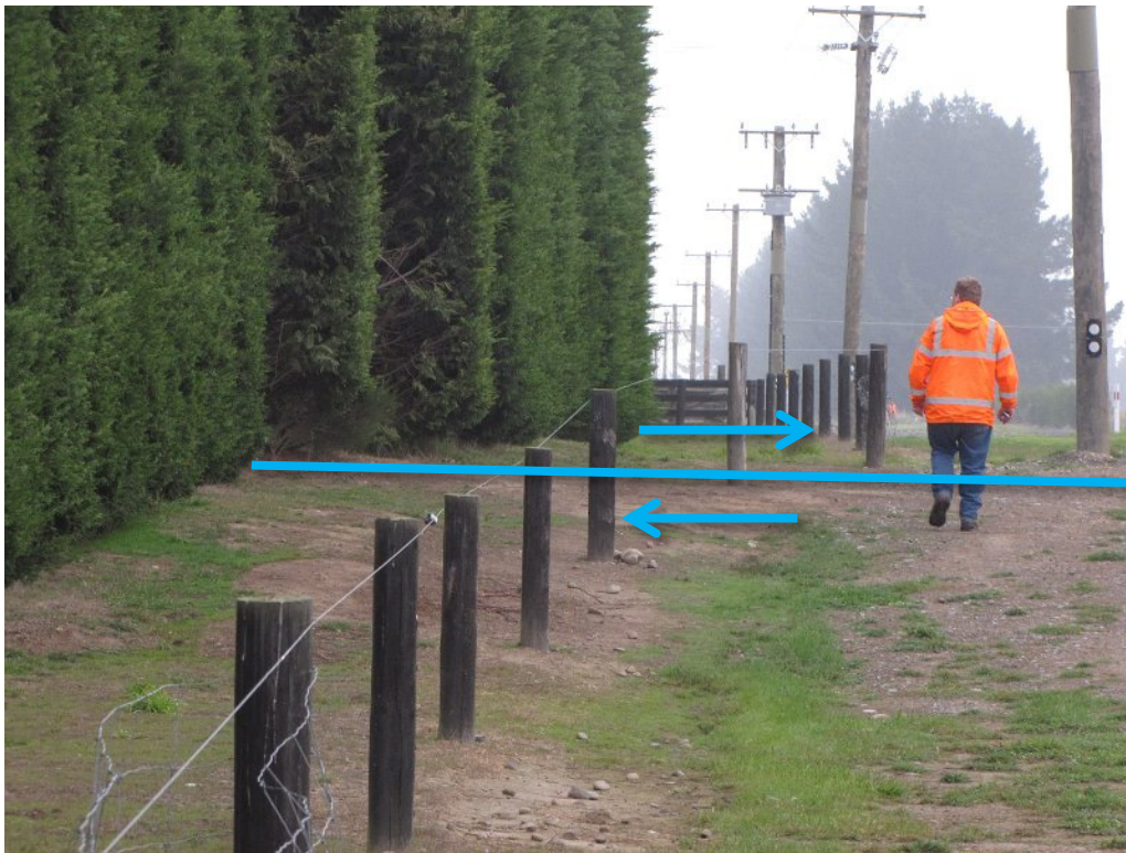
FIG. 23. Surface expression of Greendale fault, looking south. Note the formerly straight hedge and fence. Maximum offsets are 4.5 m horizontal and 1.5 m vertical.
