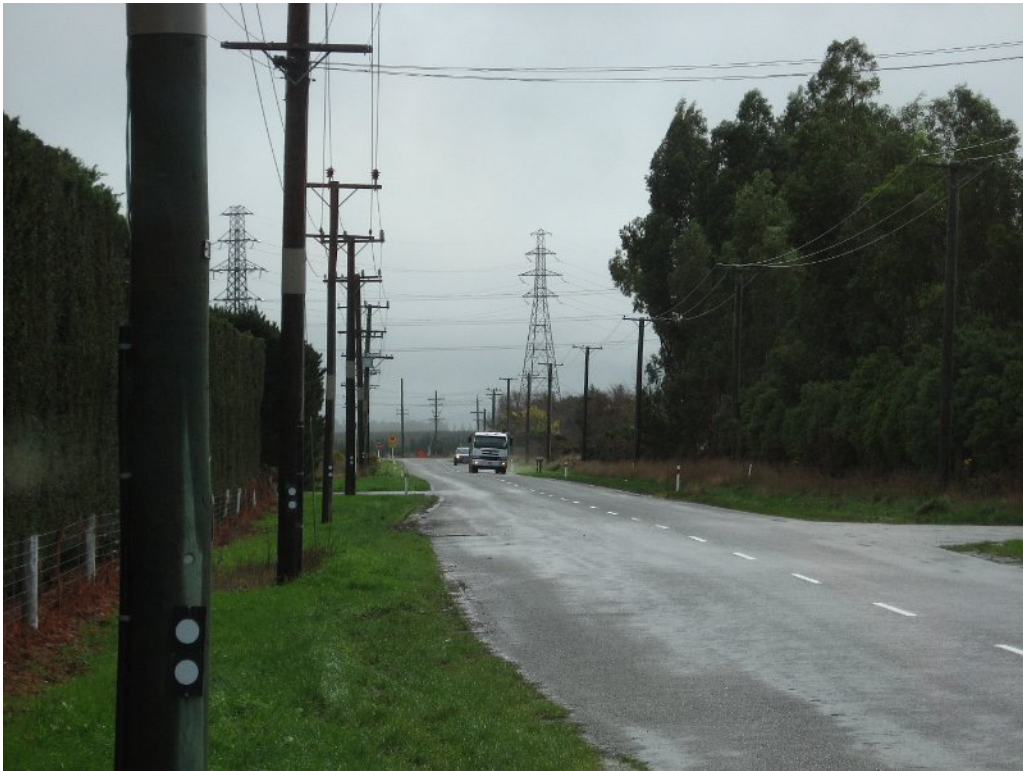
FIG. 39. Possible sources of 50 Hz power line noise (!!)
