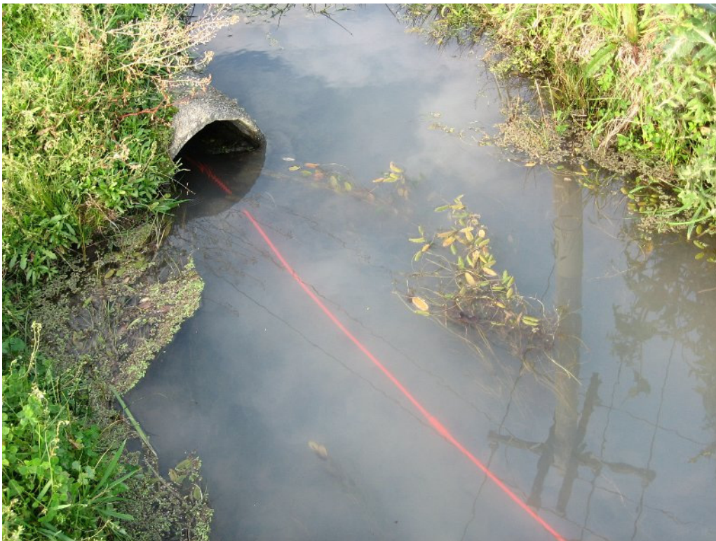
FIG. 32. Cable in a culvert. Not noisy.
