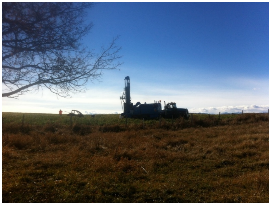
FIG. 1. Dynamite shotholes being drilled and loaded.
