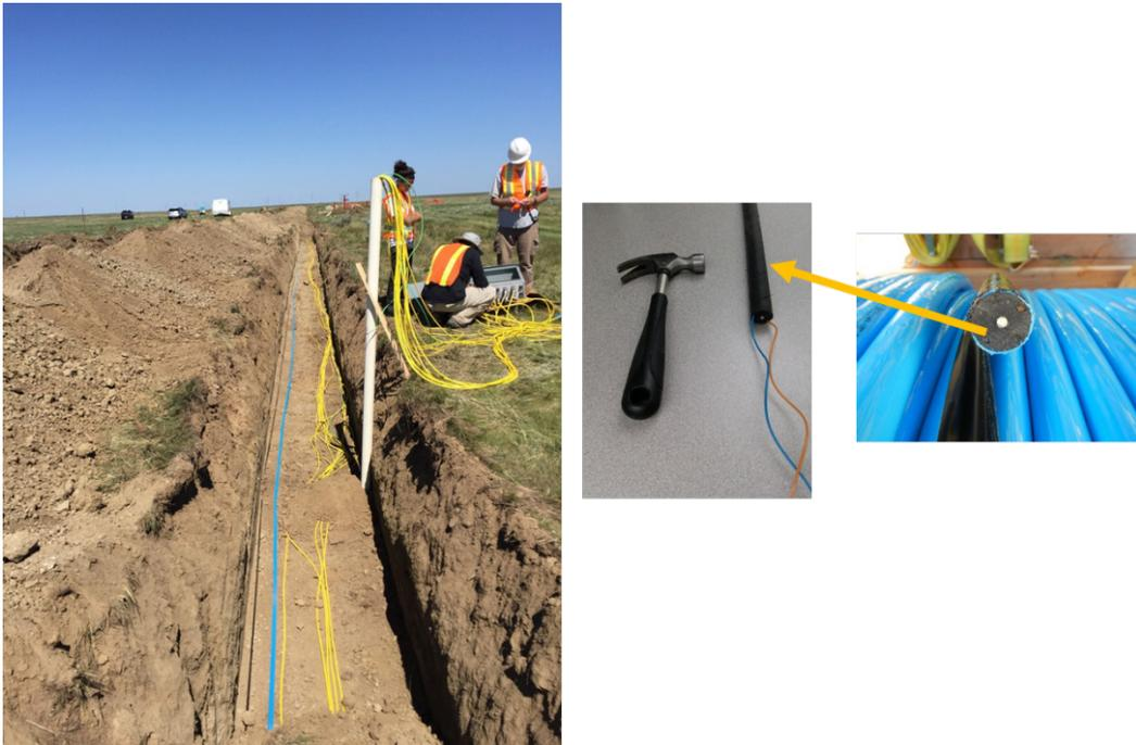
FIG 13. Straight (brown) and helical wound (blue) optical fibre cable in trench at the FRS.
