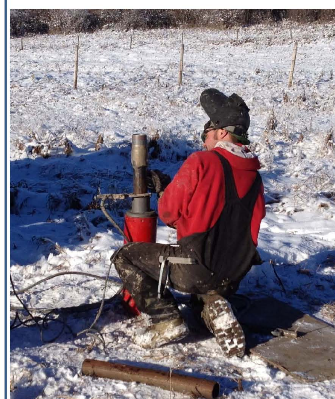
FIG 4. The bell nipple being welded onto the top of the coil tubing.
