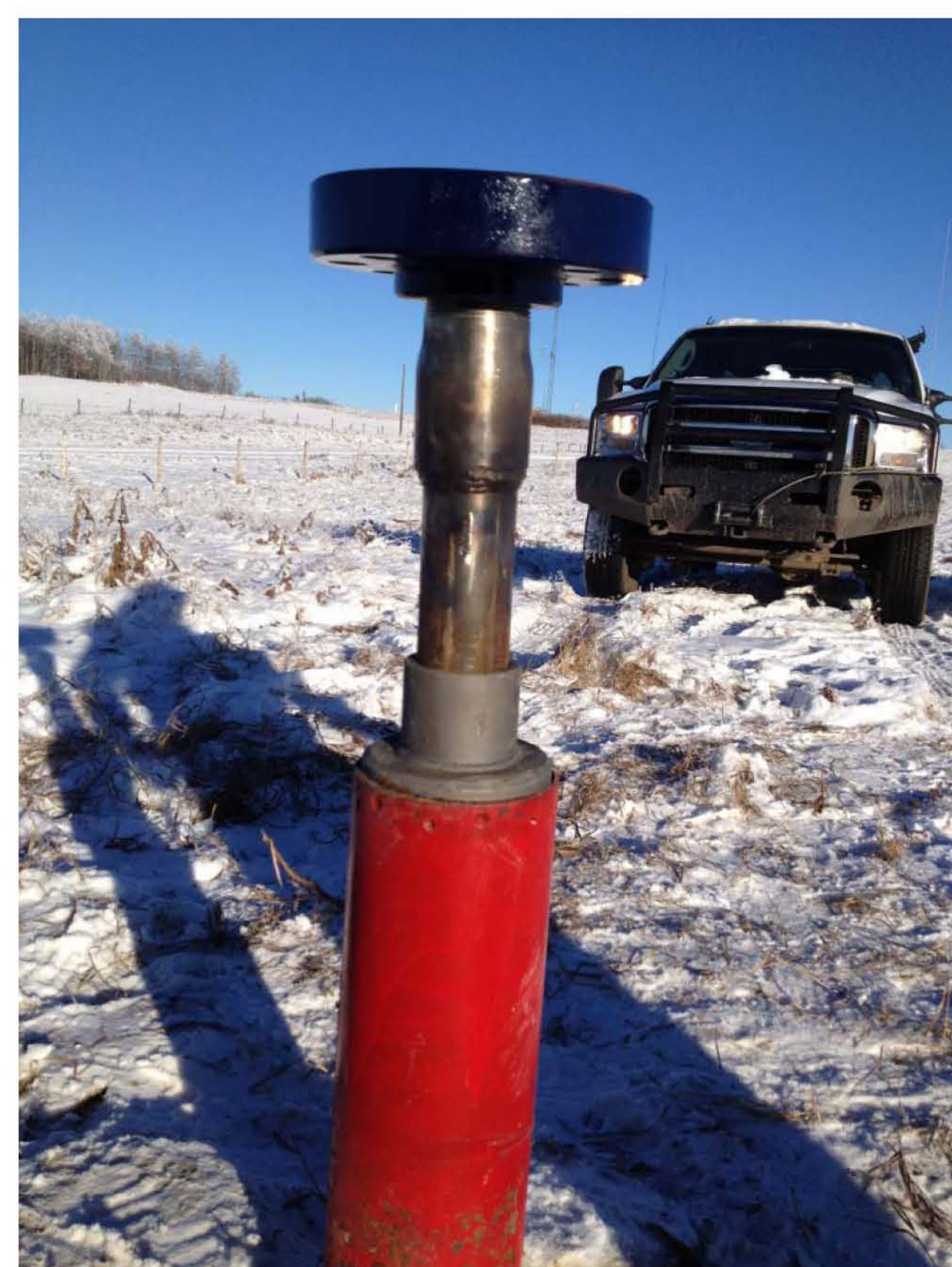
FIG 5. The finished coil tubing ready for the wellhead equipment to be installed.
