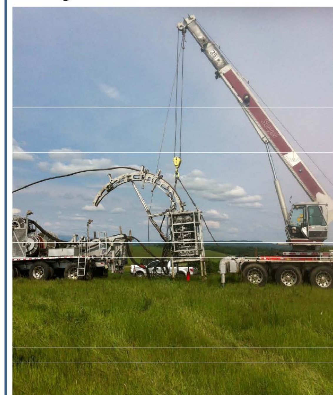
FIG 2. The coil tubing being inserted into Well 4
