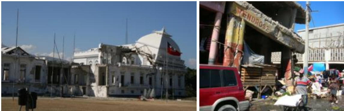
FIG. 2. The Haiti Presidential Palace (left) on January 14, 2012. The grounds have been cleaned, but the building is largely destroyed. Clean-up continues in Port-au-Prince (right). R. Stewart photos.
