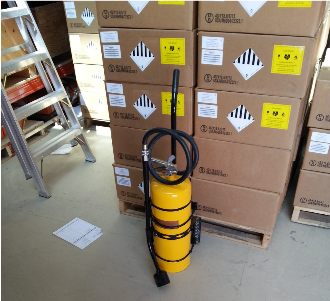
FIG. 12. The specific Class D fire extinguisher designed for lithium ion battery charging.
