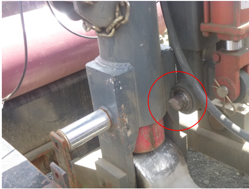
FIG. 9. The sheared off pin can be seen circled in red.
