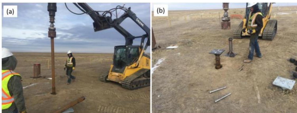
FIG. 4. Screw pile installation photos from Lawton et al. (2020). After screwing in the steel pile (a), a steel plate (b) supports small seismic sources. After the photos were taken, the pile was screwed in deeper until the steel plate was approximately 15 cm above the ground and the toe was 24.7 m below surface.
