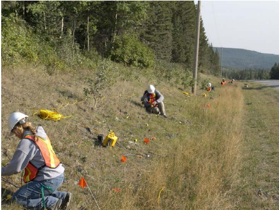
FIG. 9. High resolution spread. Geophones are located at orange flags. The Geode (yellow case) is connected to the other Geodes via a spool of yellow data cable.
