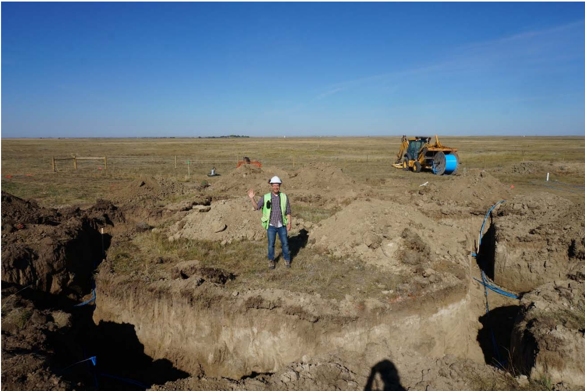
FIG. 13. CREWES Director Kris Innanen overseeing the installation of the prototype DAS array.
