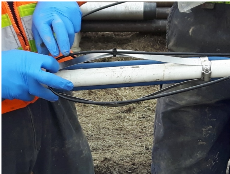
Fig. 6. Photograph showing how the DTS fiber was attached to the metal spacers to keep it flush with the borehole wall.
